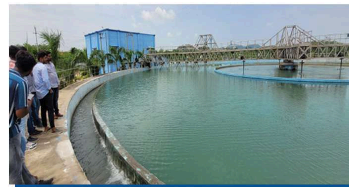
SR University Students Visit Dharmasagar Water Treatment Plant
