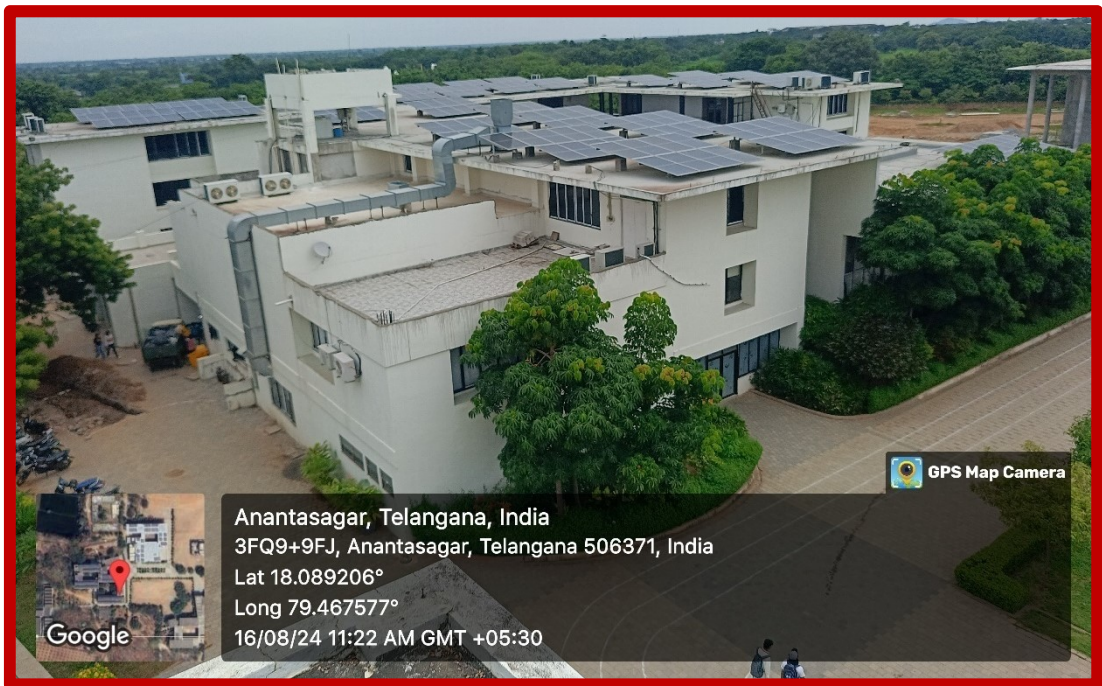
Grid-Connected Rooftop Solar Photovoltaic (SPV) Systems at SRIX
