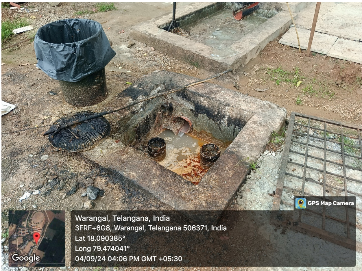
Waste Water intake Pit near the Girls Hostel
