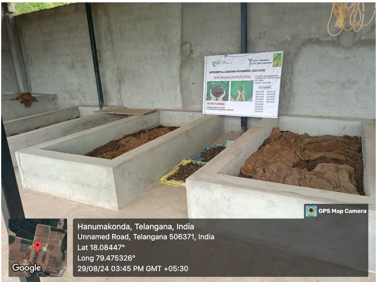
Compost Pits for maintaining the Sludge
