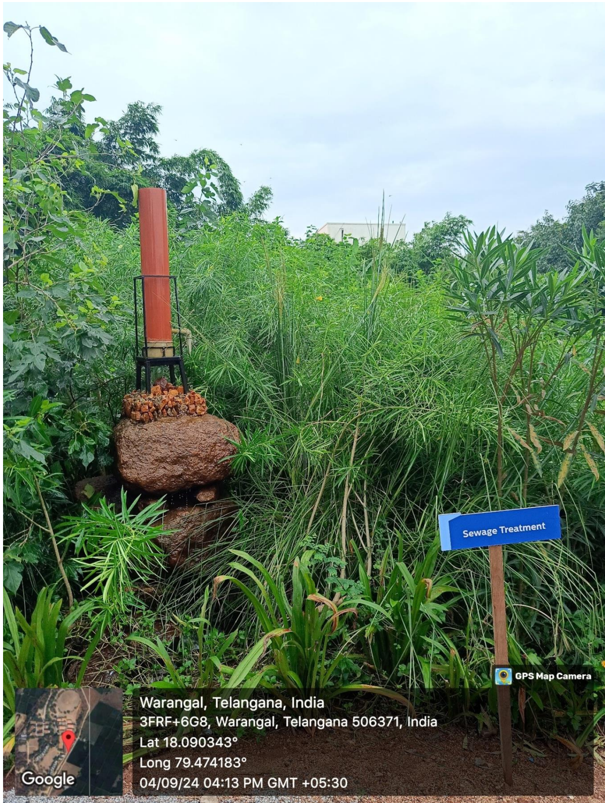
Reed bed system for Sewage Treatment
