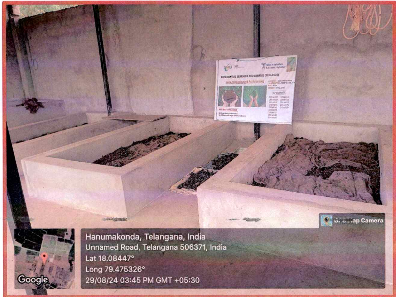
Compost pits for maintaining the sludge
