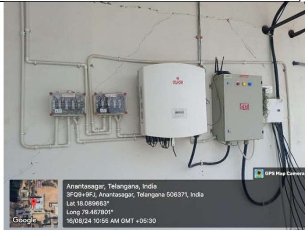
Connecting the Solar power to the Grid
