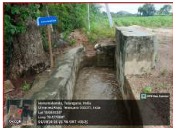
Rain water surface canal towards water bund
