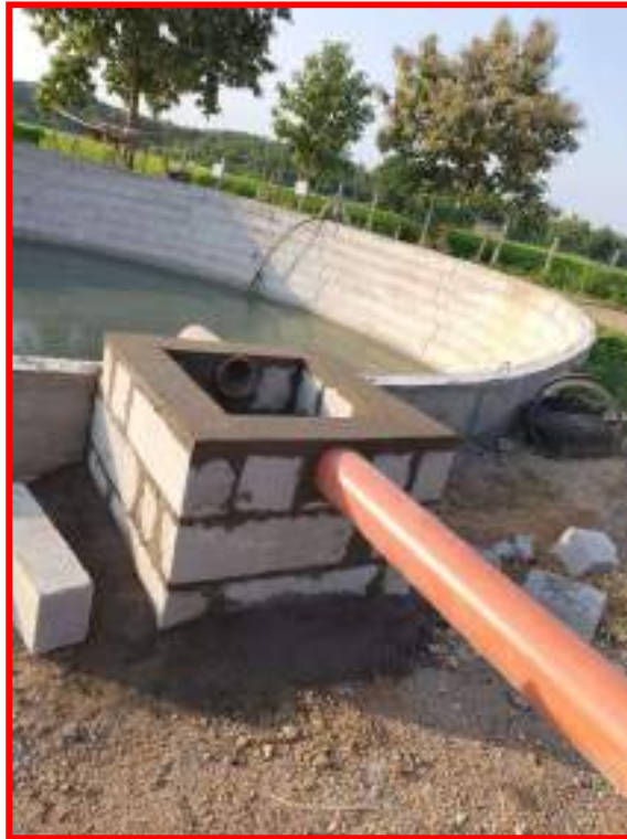
Open Well Recharge near the Security Check Post
