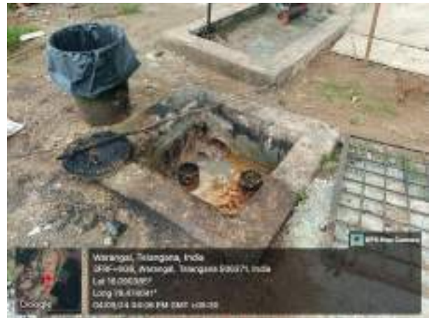
Waste water intake pits
