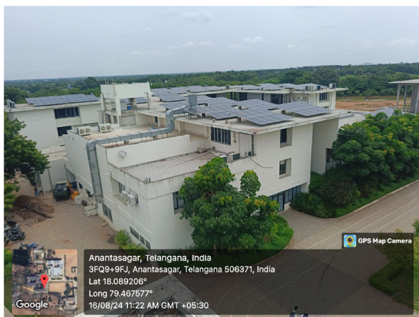
Solar Panels at SRU
